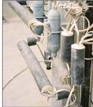
✗ Unsealed bundle ends, splices and terminations allow moisture to be absorbed by the insulation. Wet insulation degrades the bundle two ways: by reducing the insulating properties and secondly by releasing water soluble chlorides which may contribute to chloride stress corrosion of stainless steel process tubes.
