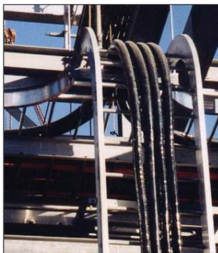
✓ O'Brien's TRACEPAK® has a unique design which allows for an 8" (203mm) bending radius.
