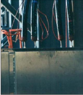
✗ Leaving several inches of tubing exposed at the end of a tubing bundle leaves the entire system open to freezing. Stainless steel tubing can lose more than 100°F (38°C) per inch if not insulated and traced.
