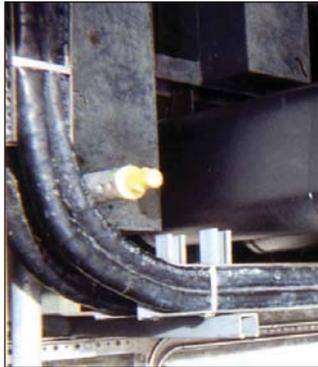
✗ When supporting tubing bundle in a cable tray, care should be taken to keep bundles from touching each other. Supports and hangers must have a large surface area and be designed so they can not be overtightened to crush the tubing bundle.
