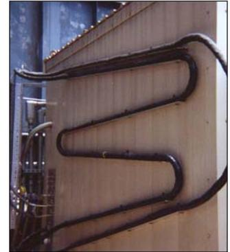
✗ When using MI heater cable or other heaters that cannot be cut to length accurate measurements of the sample line length are critical. Sample bundle must be installed so that there is a continuous slope toward the sample system.
