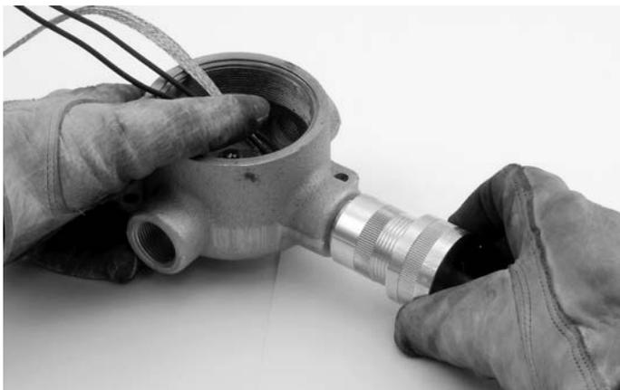
18. Install the bus wires into the Item 15 TERMINAL BLOCK. If the application is an end connection, stow the block inside the junction box and connect the braid pigtail to the grounding lug in the junction box.
