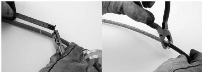
6. Lightly crimp on item 8 LEAD WEDGE. Do not use excessive crimping action distorting the wedge. Locate the wide side of the taper of the wedge at the end of the jacket. Insure the wedge does not cover any portion of the jacket material and is covering only the braid.
