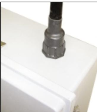
**✓** Bringing the insulated tubing bundle in to the cabinet through a weatherproof entry seal to maintain the integrity of insulation and heating in tubing bundles.
