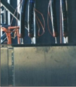
**X** Leaving several inches of tubing exposed at the end of a tubing bundle leaves the entire system open to freezing. Stainless steel tubing can lose more than 100°F (38°C) per inch if not insulated and traced.
