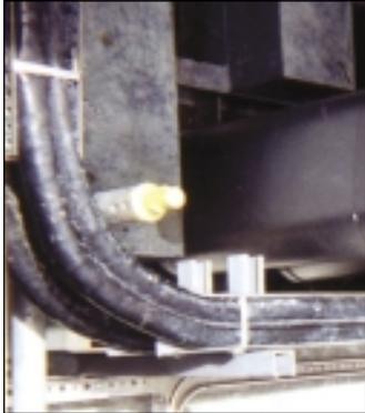
**X** When supporting tubing bundle in a cable tray, care should be taken to keep bundles from touching each other. Supports and hangers must have a large surface area and be designed so they can not be overtightened to crush the tubing bundle.
