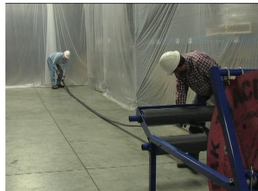
With a steady motion, pull bundle through roller assembly. Continue to pull bundle through rollers to desired length.
