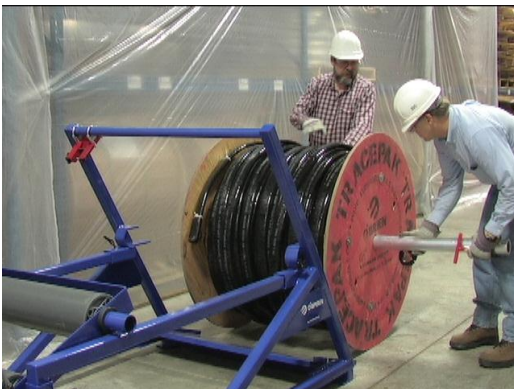
Insert shaft through spool and install collars.
