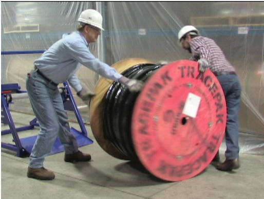
Rotate spool so bundle comes off the bottom.
